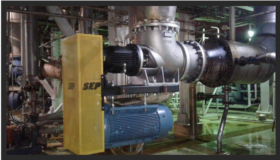
PAKMAYA (KÖSEKÖY) SEP GEP SERIES AXIAL FLOW PROPELLER ELBOW PUMPS (YEAST PRODUCTION PLANT)
