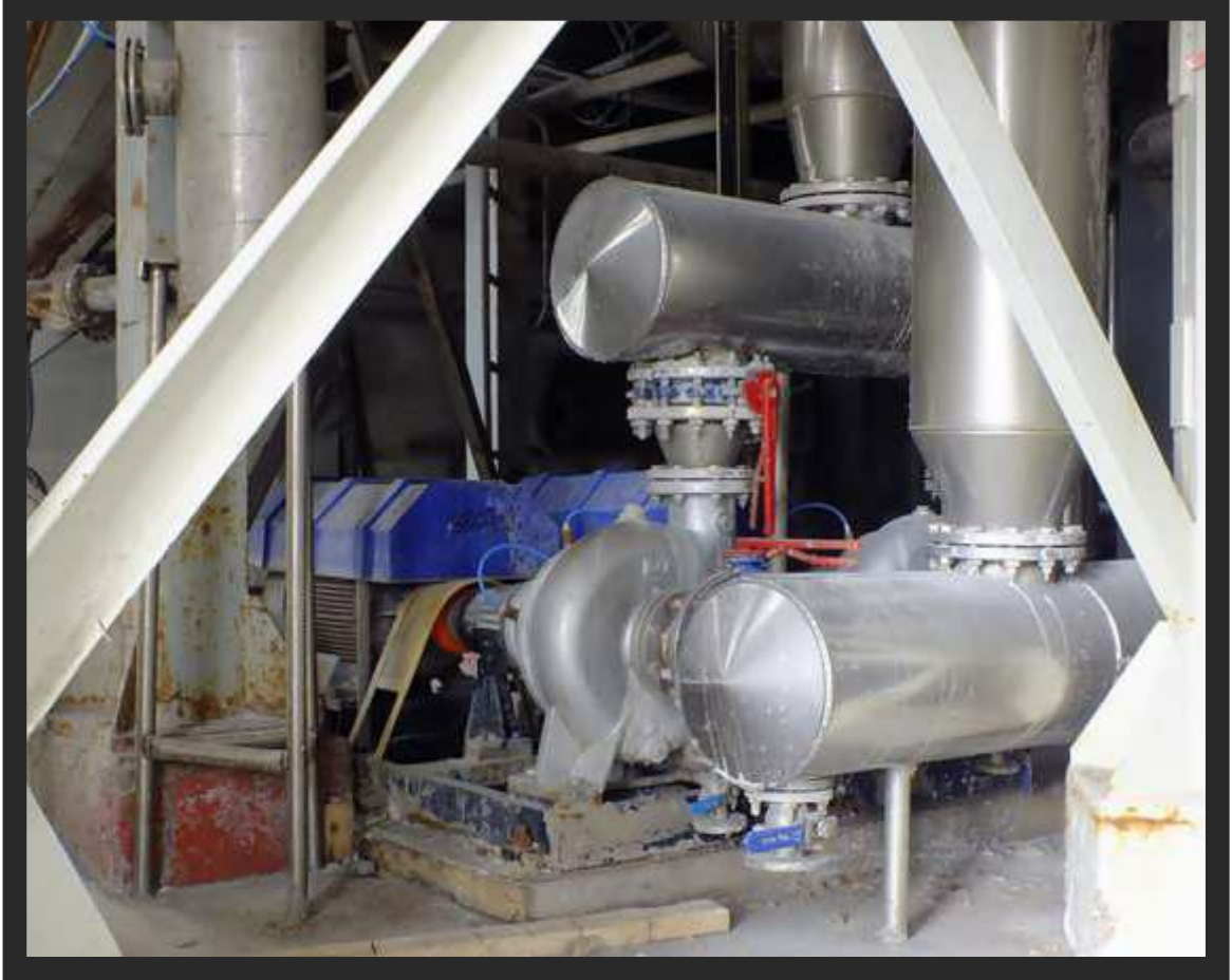
BİLLURTUZ (İZMİR) SEP GP SERIES PROCESS PUMP (REFINED SALT)
